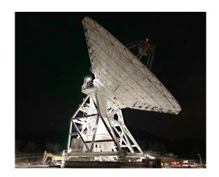
Is largely done by a Satellite dish antenna DSS-42 built in 1965 and located in Australia. It has a 26 meter in diameter.
